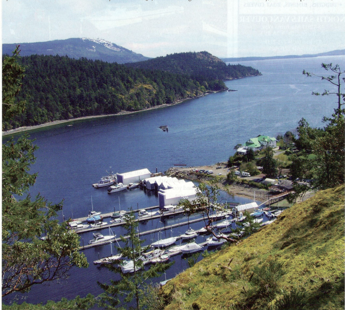
[Above] The entrance to Genoa Bay is well marked by day markers on each side.
